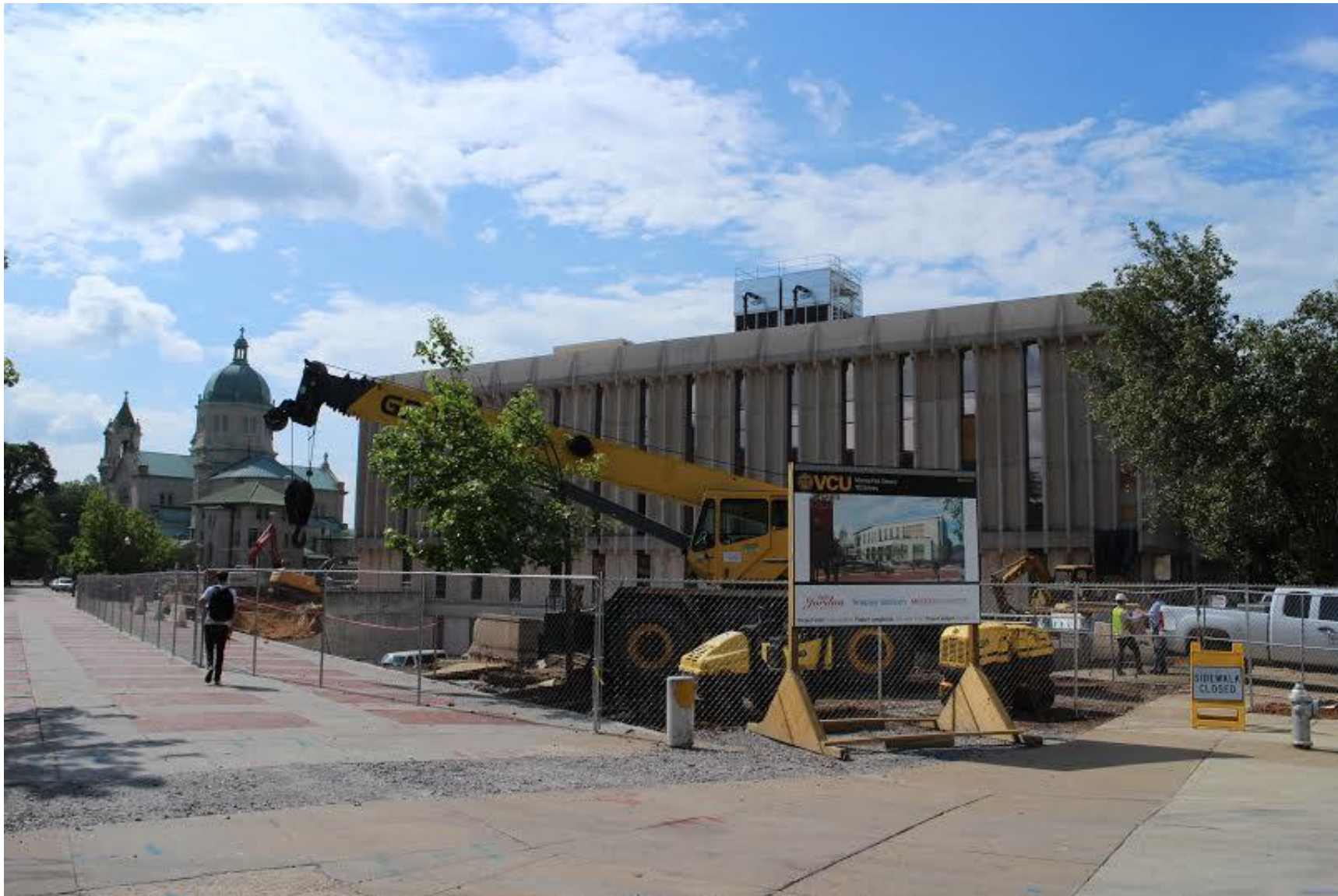
Cabell Library under Construction (Photograph by Brandy Brubaker.)
